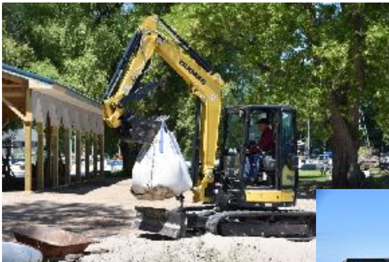
Sand Bags re-used
